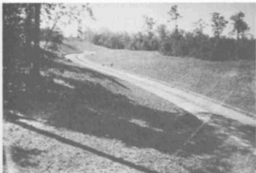
Biltmore entrance drive under construction, ca. 1890s. (Courtesy National Park Service, Frederick Law Olmsted National Historic Site)
